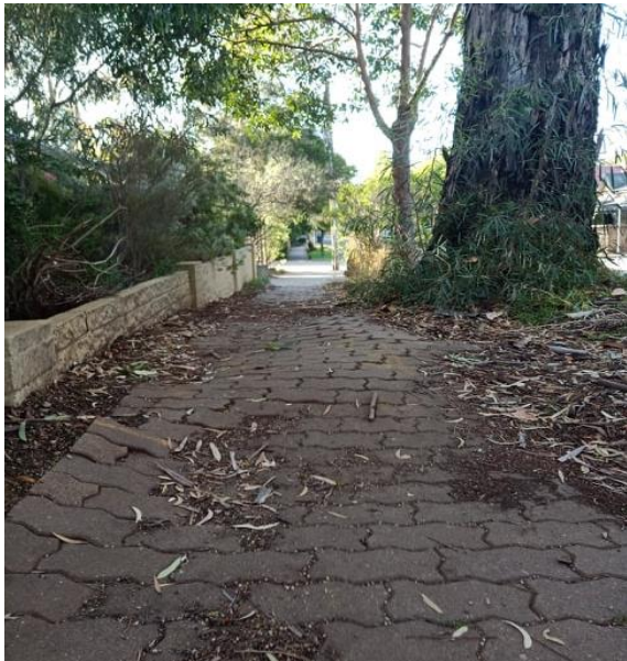
Figure 2.7: Footpath along Gilbert Street
